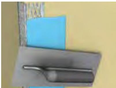
Using a 4" broad knife, apply setting compound to the bead to a width of approximately 4" each side of the corner, filling all perforations.
