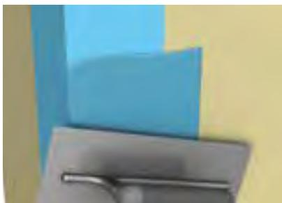
Apply second coat to a width of approximately 120mm. Allow to dry, then remove any excess and lightly sand if necessary.
