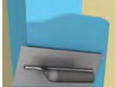
Apply third coat with a 8" broad knife. Feather edges with a wet paint brush. Allow to dry.
