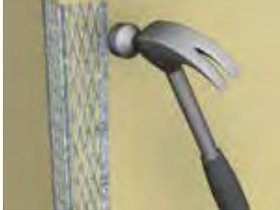
Beads can be attached by nails or a staple gun at not more than 500mm centres down the legs of the bead, and not more than 4" from each end.
