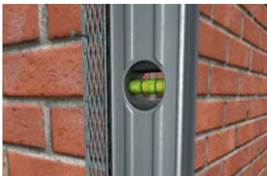
■ ENSURING THE BEAD IS PLUMB AND STRAIGHT
