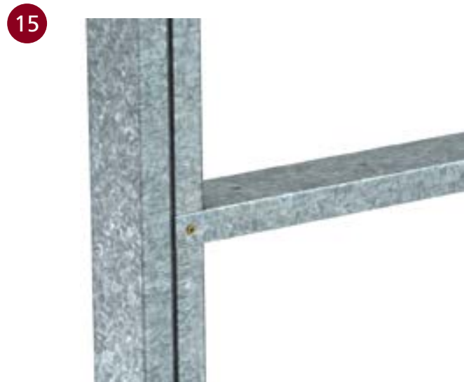
■ NOGGING TRACK FIXING DETAIL AT MAXIJAMB
